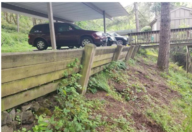
Retaining Wall-Wood
