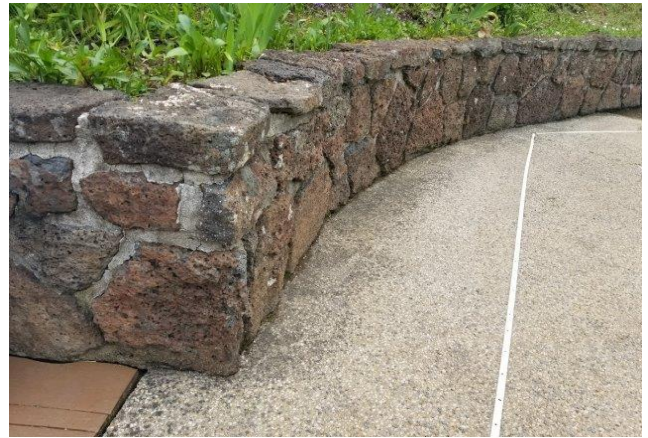
Pool-Retaining Wall-Lava Rock
