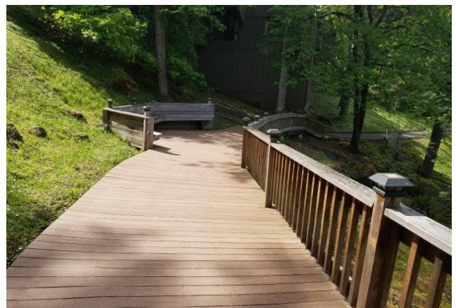
Walkway-Composite-Top Boards
